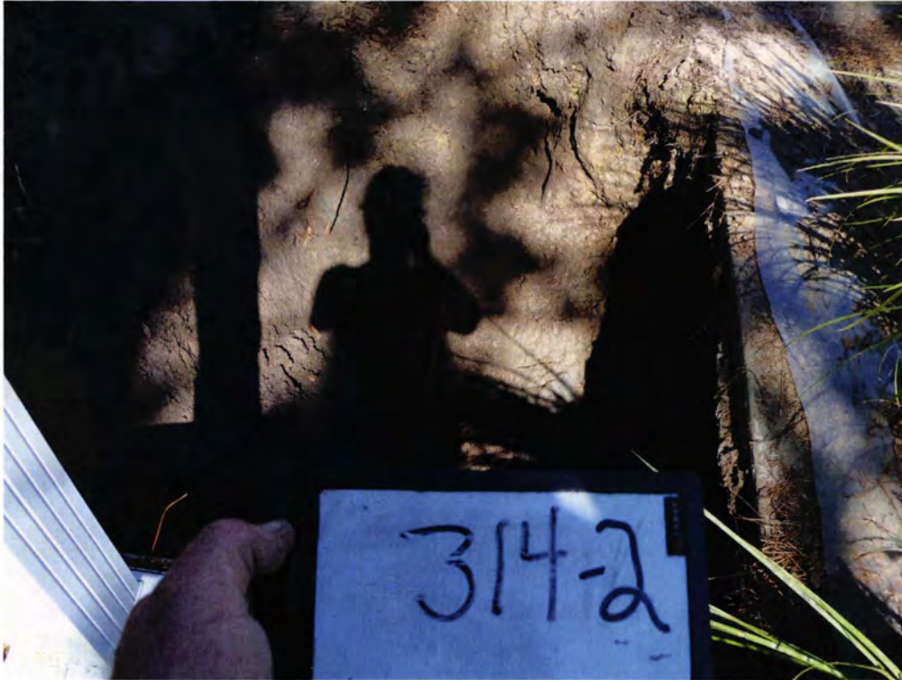
Picture 3: UST 314 Ash-2 excavation.
