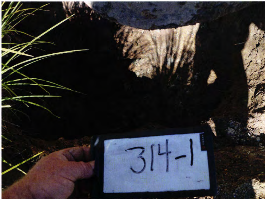
Picture 2: Excavation of UST 314Ash-1.
